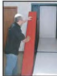
2) When unit is stable in the 'tee-pee' position face the cabinet. Push unit toward cabinet with lower hand while stabilizing with other hand until top engages with cabinet top locks.
